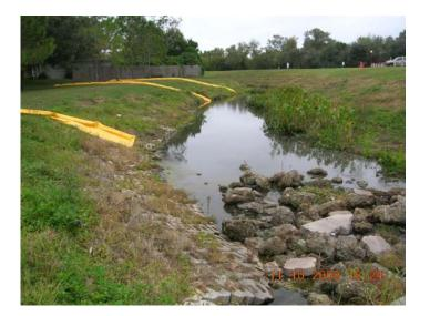
These barriers will not prevent downstream sedimentation with this installation...Even if placed in the stream, turbidity curtains cannot stop downstream sediment transport if there is a significant flow velocity.
