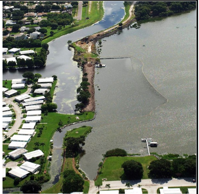
Figure 5. Alum facility on Lake Seminole during construction
