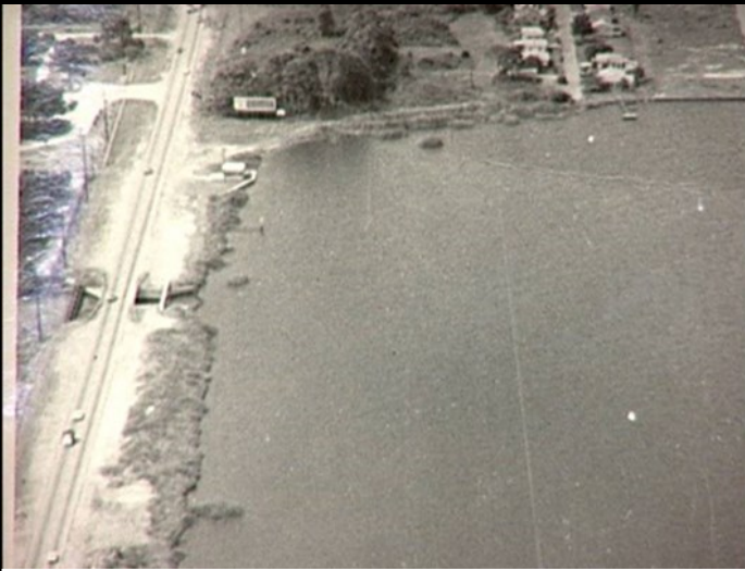
Figure 2. Lake Seminole Outfall during Construction of lake
