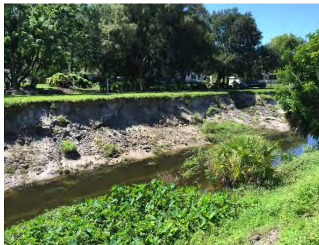
Figure 2.2 Joe's Creek Bank Failure
