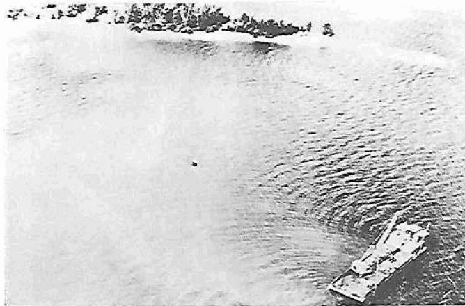
Figure 11. Open water disposal of maintenance spoil from berths in Hillsborough Bay into submerged spoil area behind an existing spoil island, December 1973.
