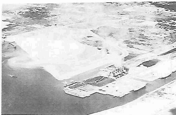
Figure 7. Deepening of East Bay (Upper Hillsborough Bay), September 1967. Material dredged was used to fill in submerged land and mangroves for a phosphate loading port facility.
